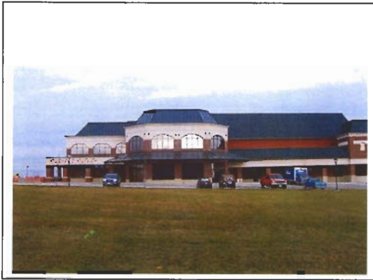
▲ This Movie theater at Maple Tree Place (Williston, VT) is an example of a large-scale project that features a hipped roof..
