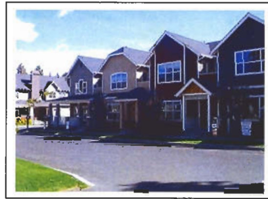
▲ This townhouse development (Bend, OR) features a varied roofline, incorporating both traditional front-gable as well as hipped gables.
