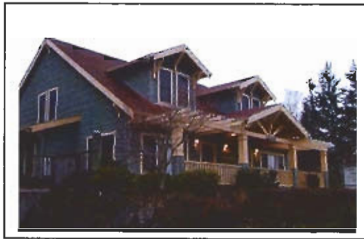
◀ The steeply pitched side-gabled roofline with dormers of this office commercial building (Clackamas County) is varied, as well as interesting to look at and is evocative of the Craftsman Style.
