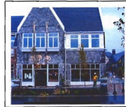
▲ Lakeview Village (Lake Oswego) uses rusticated stone as the primary building material for this portion of the office retail development.
