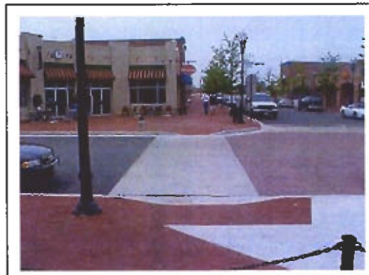
Textured Sidewalks and Crosswalks
