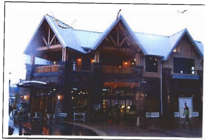
▲ The Lakeview Village development (Lake Oswego) is an example of a large-scale retail project that incorporates a varied roofline using steeply-pitched, front gables.
